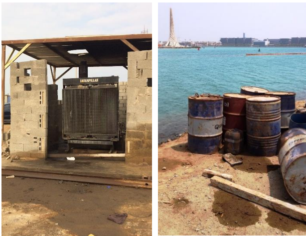
Generator fuel spillage and oil drum storage non-compliances
